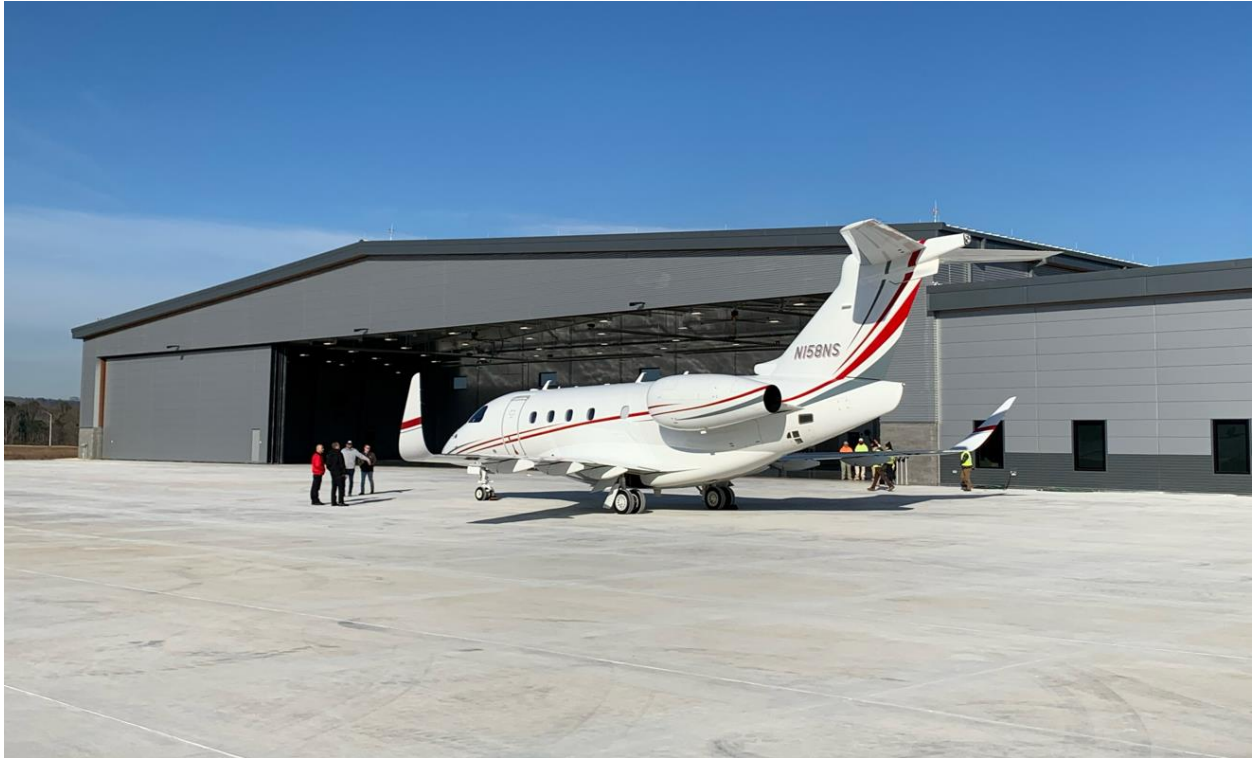
Figure 2-13: Norfolk Southern Corporate Hangar (North Terminal Area)
